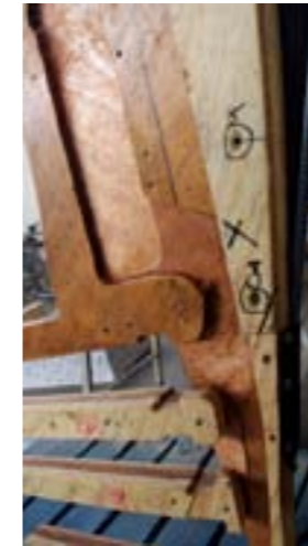
Cut out for the cable routing
